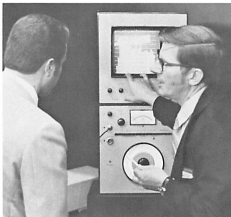
Roy Nelson (r), supervisor for CPD's engineering and R&D, presents an interesting evaluation of the frequency response range of Memorex audio tape to a CES visitor. The presentation was made by means of a real time analyser, which can display the frequency response range of any audio tape and compare frequency characteristics of competitive tapes.
