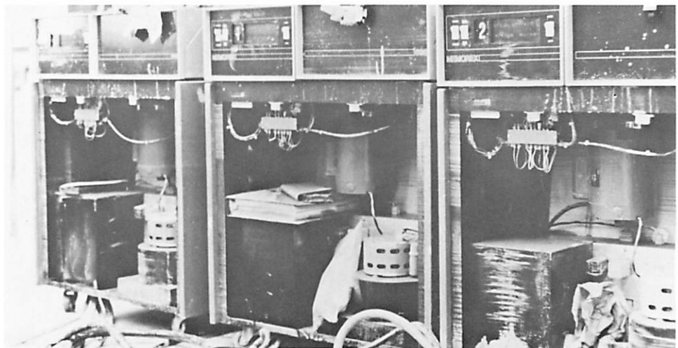
Caked with mud and silt, these 630's were in four feet of water when tropical storm Agnes
