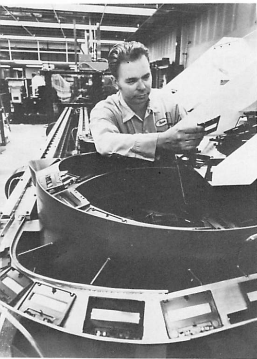
Mechanic Norm Kahr checks a few of the cassette shells being fed into the giant Rockford #2.
