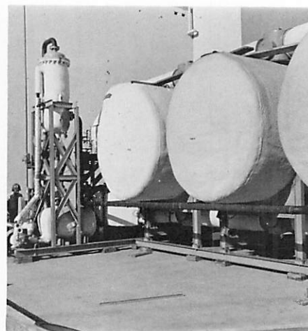
Audio tape plant's solvent recovery system
