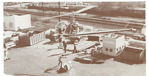
The people shown on page 3 were watching this helicopter lift some heavy air conditioning equipment onto the plant roof a couple of weeks ago.
